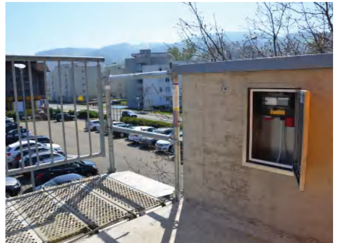
Unobtrusive recessed distribution box
