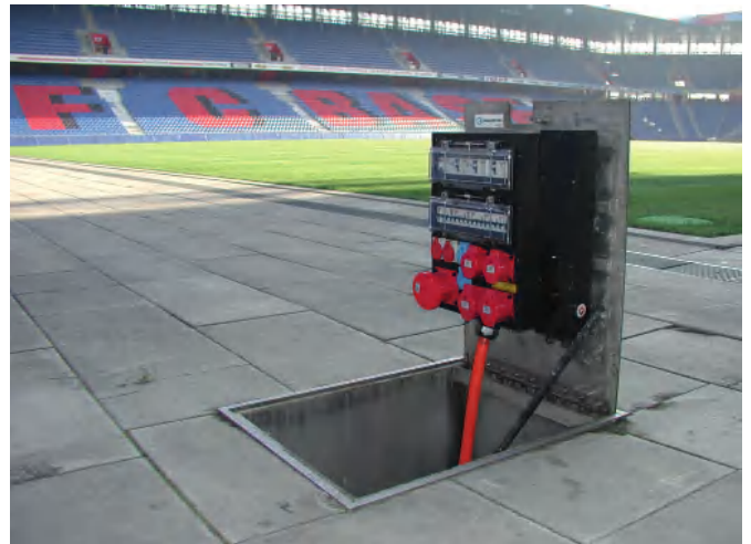
Underfloor distributor system, St.Jakob-Park stadium in Basel
