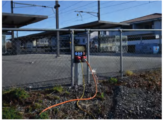
Power distribution box at Oberriet railway station
