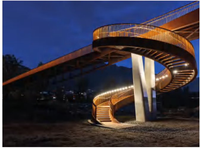
LaneLED WALL, Torretta Bellinzona footbridge
