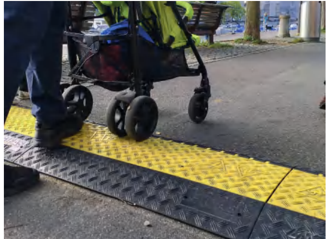
Cable crossover in Zurich
